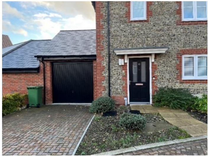
Fig 67. Somerset Field property with flint elevations
