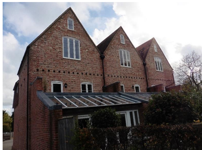
Fig 36. The renovated oasts houses at Holmes Field Court
